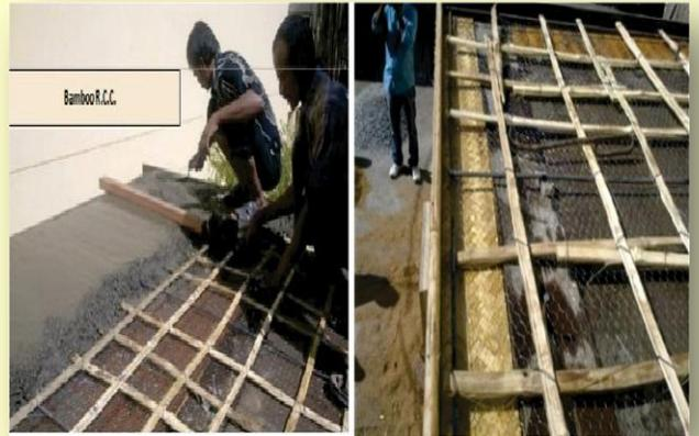
*Construction at IPIRTI, Bangalore with Bamboo reinforcement*
