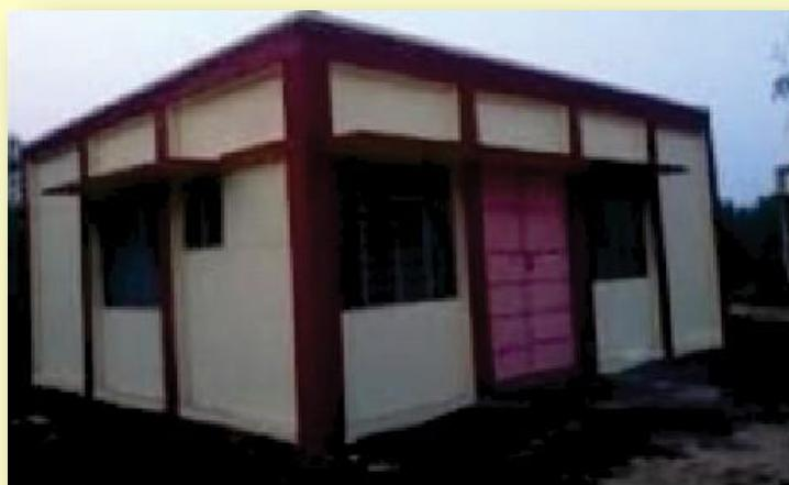
**Fig. 2 : A model 2 BHK bamboo reinforced concrete house constructed in school premise near IIT in 2014**
