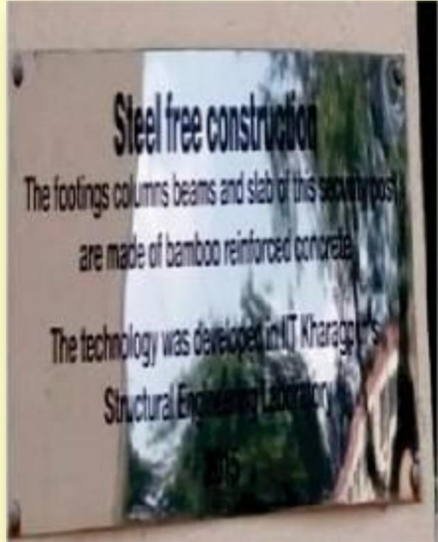
**Fig. 4 : Plate in the house mentioning STEEL free construction**
